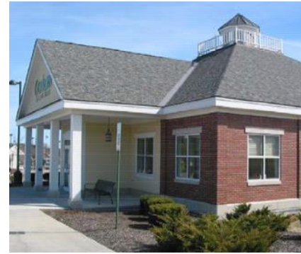
fig 10.1: Effective use of materials & detailing. Inappropriate scale and use of ventilation cupola & railing.
