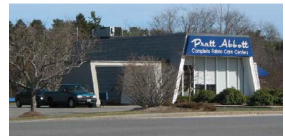
figs 9.2 & 9.3: Inappropriate Structure Forms
