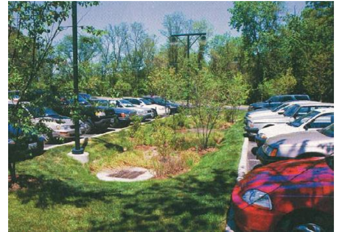
figs 5.2 & 5.3: Parking Integration into Natural Landscape; Stormwater Bioretention
