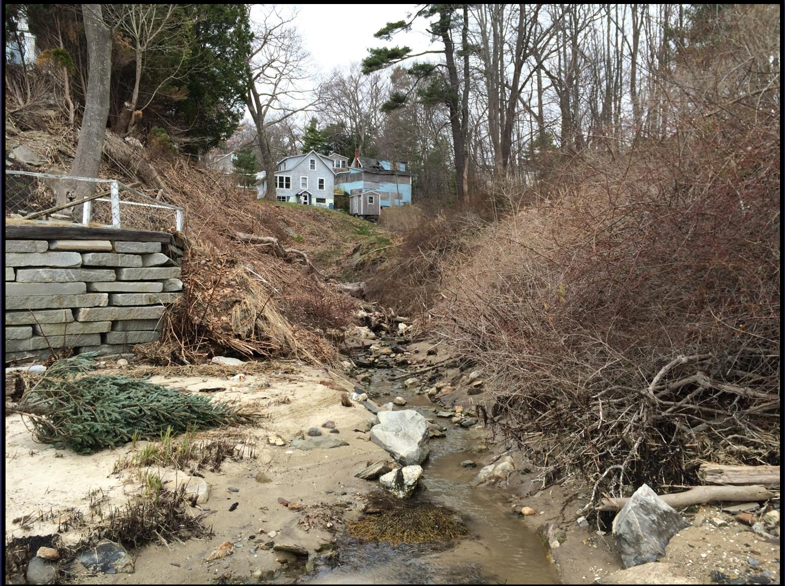
5. 2015 Drainage Channel looking upstream from beach
