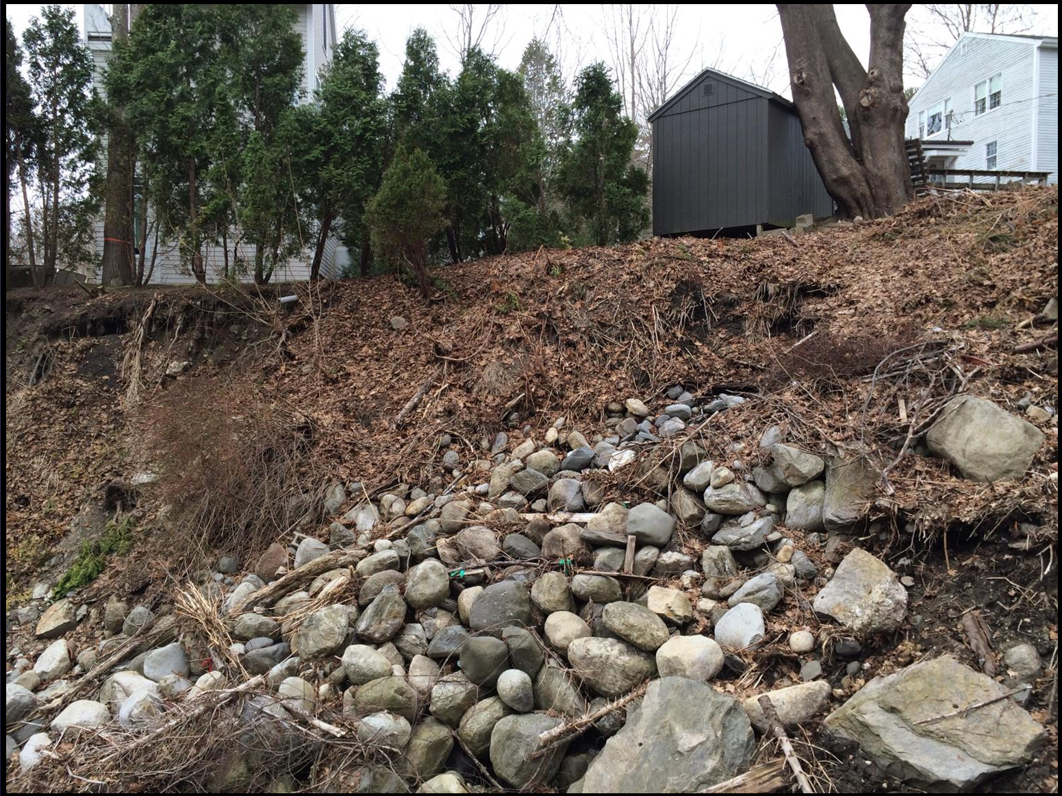
5.2015 Existing Riprap Apron at Outfall
