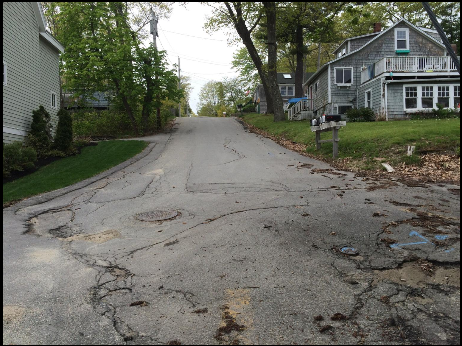
5.2015 View from Base of Underwood Road
