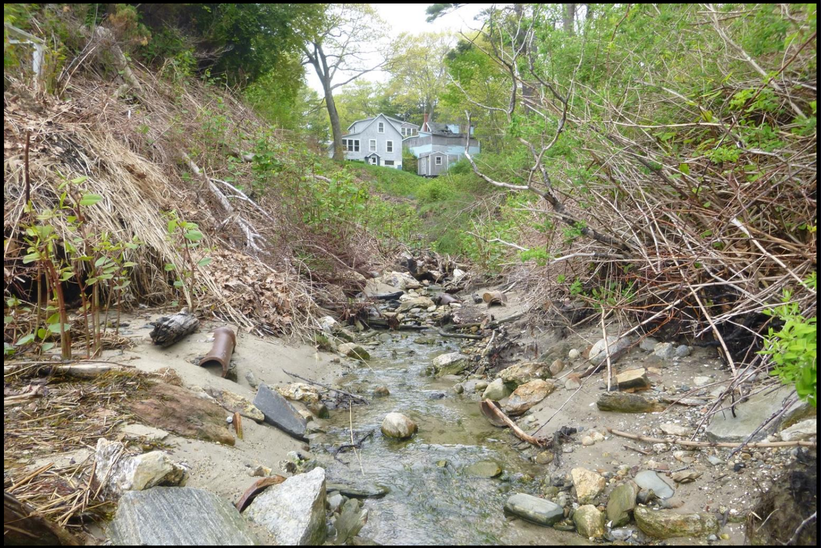
5.2015 Drainage Channel looking upstream to Stormwater Outfall (2)
