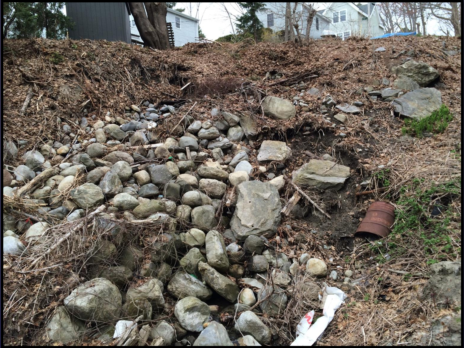
5. 2015 Stormwater Discharge Outfall
