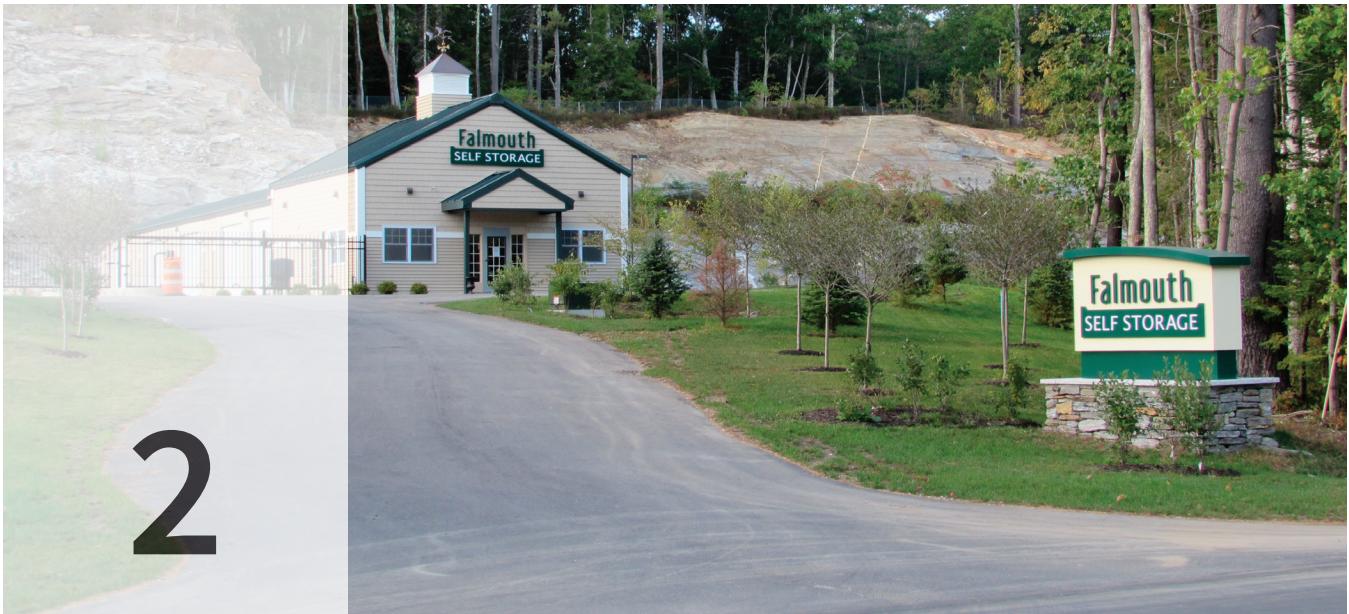
Existing Building, Route 1 North, Falmouth
