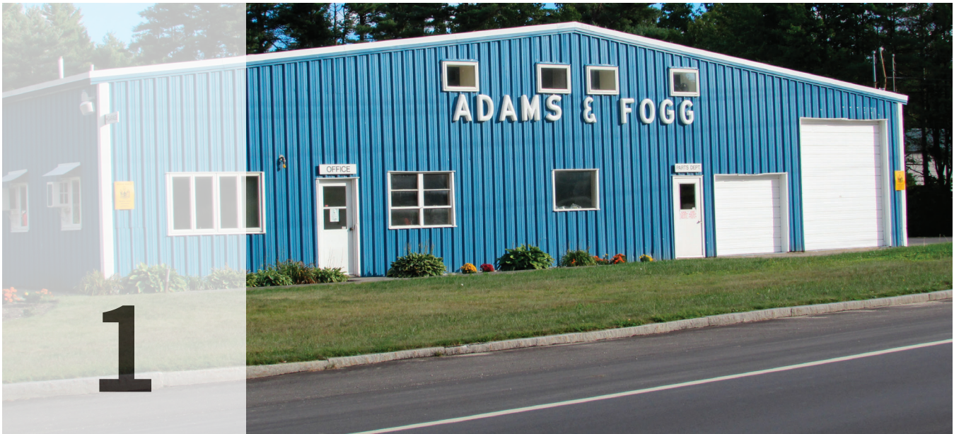
Existing Building, Route 1 North, Falmouth
