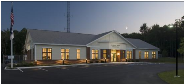
Figure 8: Police Station, Marshal Drive
