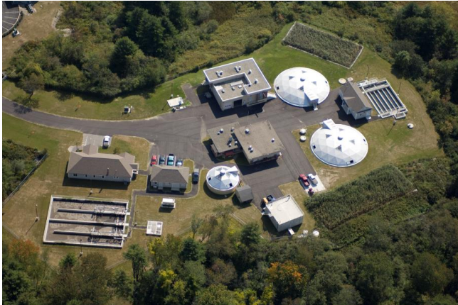
Figure 9: Richard B. Goodenow Wastewater Treatment Facility
