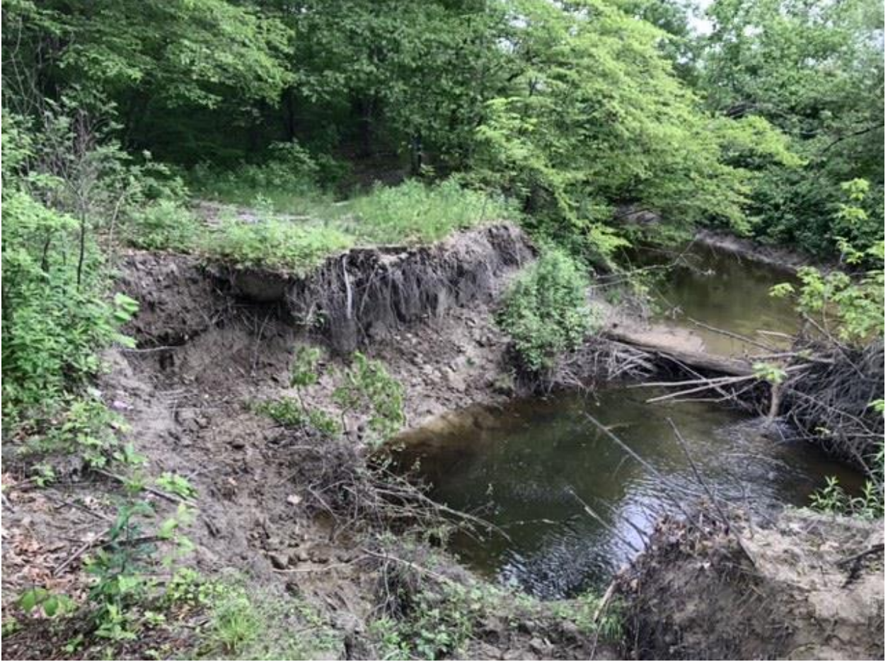
West Branch Erosion Damage
