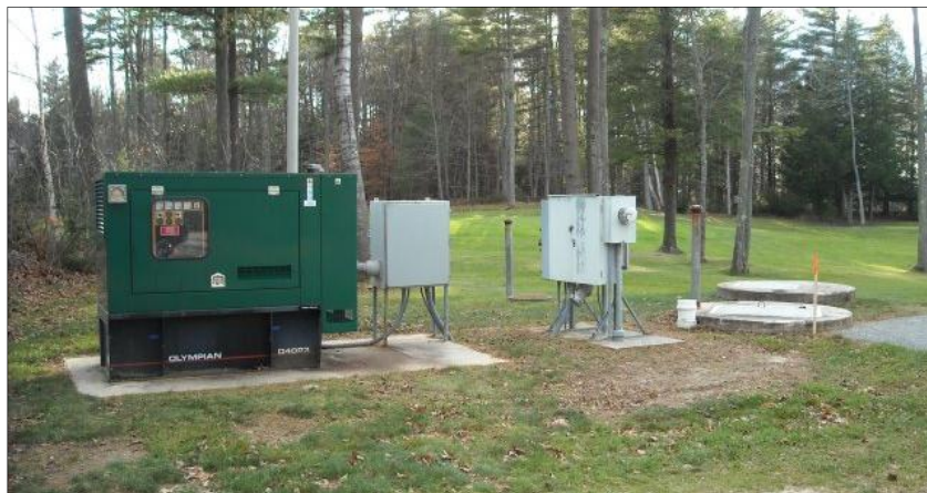
FIGURE 2-6 PINEHURST DRIVE PUMP STATION
