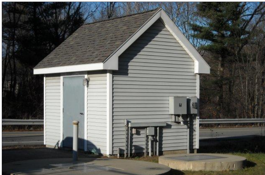
FIGURE 2-10 LEIGHTON ROAD PUMP STATION
