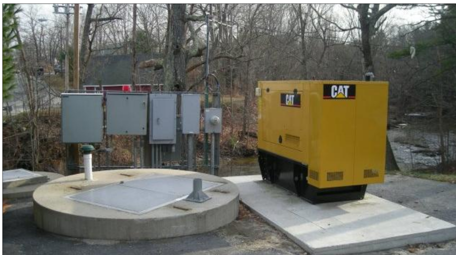
FIGURE 2-11 MILL ROAD PUMP STATION
