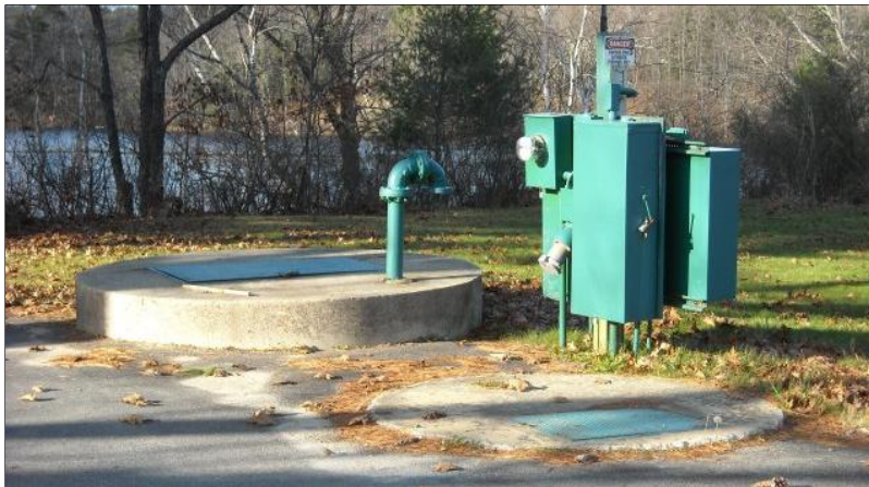
FIGURE 2-4 MIDDLE ROAD PUMP STATION
