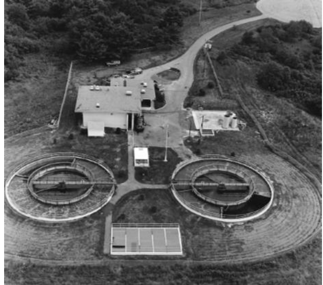
Aerial view of the new treatment plant in 1970
