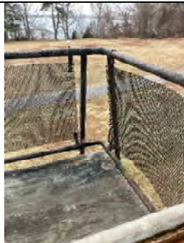
Steel and Plywood Balcony.
