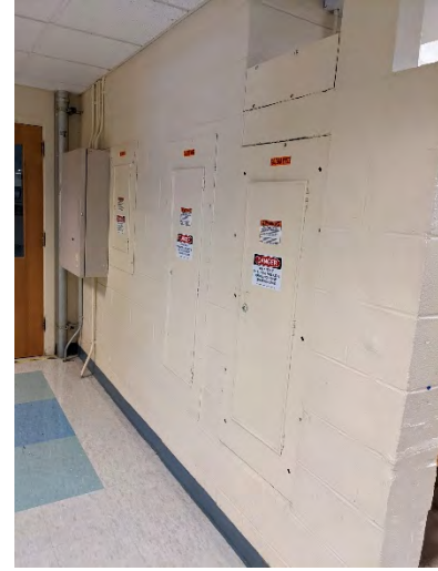
Ex. Inaccessible Panels Serving Kitchen
