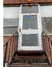
Exterior exit stair.
