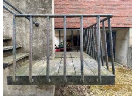
Exterior stair detail
