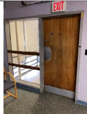
Typical interior condition
