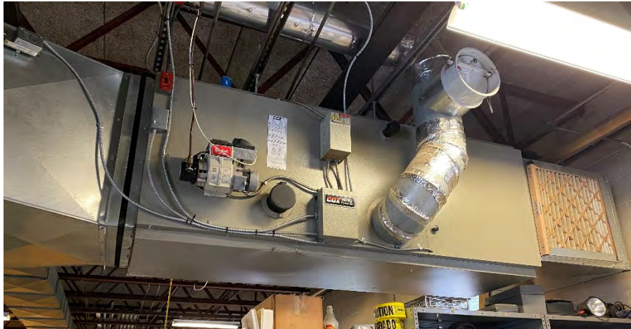
Figure 3 - Oil-fired Furnace
