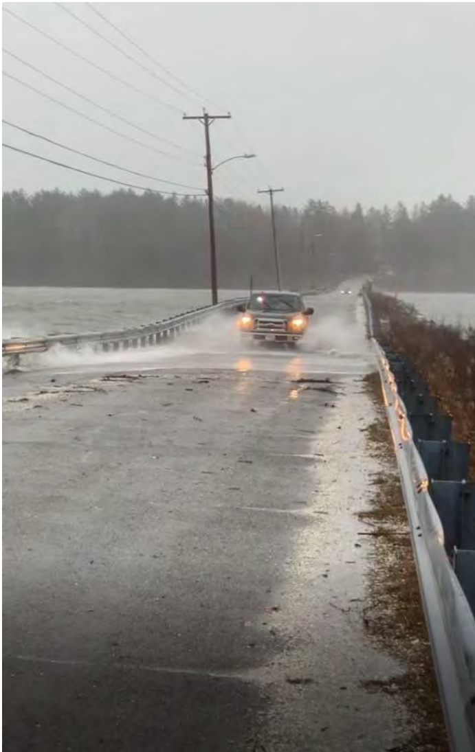
Fig. 1. Causeway Overtopping During December 23, 2022 Storm Event
