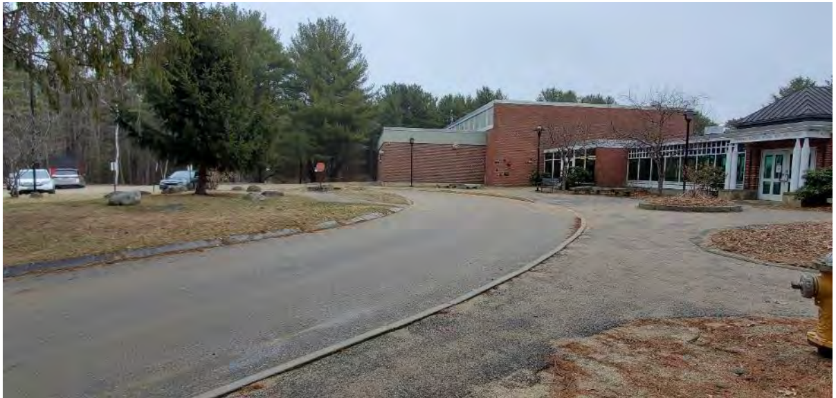
Photo 10: MECDHH Main Entrance
