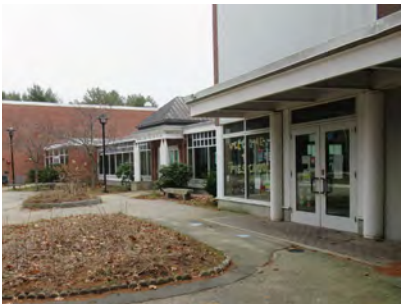
MAIN SCHOOL ENTRY
