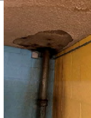
Roof leak.
