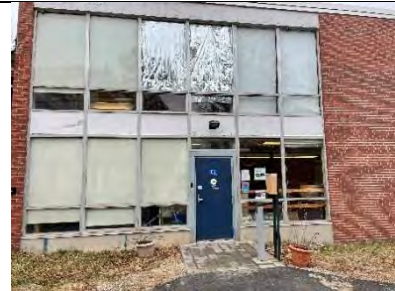
Existing Aluminum Curtainwall.
