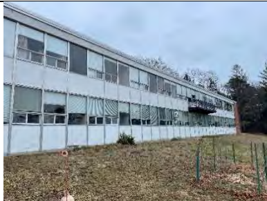
Existing Aluminum Curtainwall.
