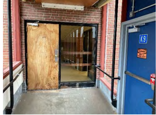
Interior at door to Building K.
