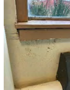
Existing window sill.
