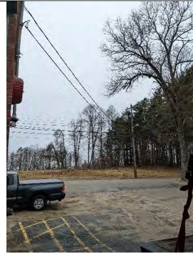
Incoming Overhead Power
