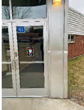
Damaged siding.
