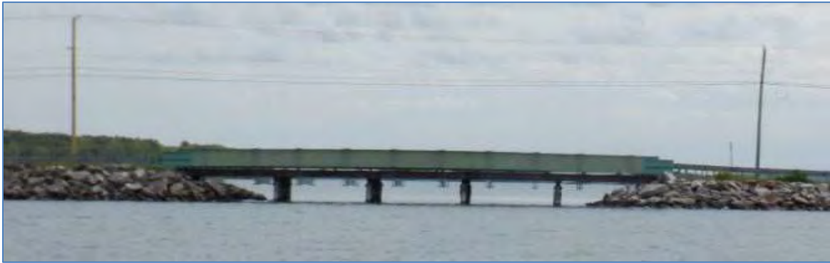
Fig. 9. Mackworth Island Bridge Looking East from Boat
