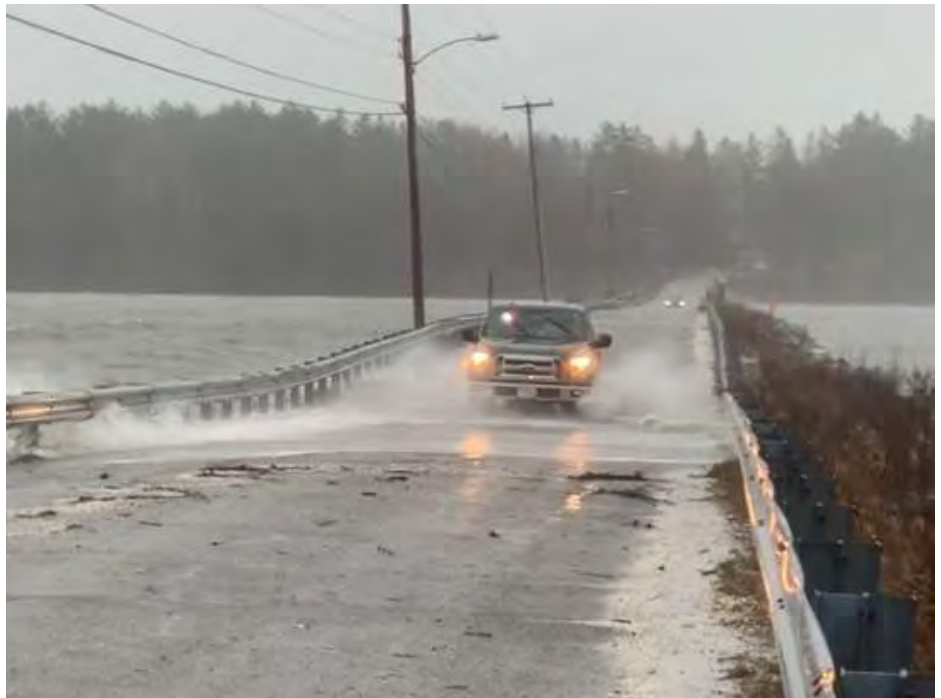
CAUSEWAY OVERTOPPING DURING DECEMBER 23, 2022 STORM
