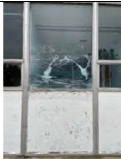
Exterior siding/glazing system
