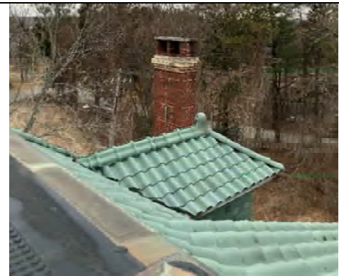
Roof tile & EPDM.
