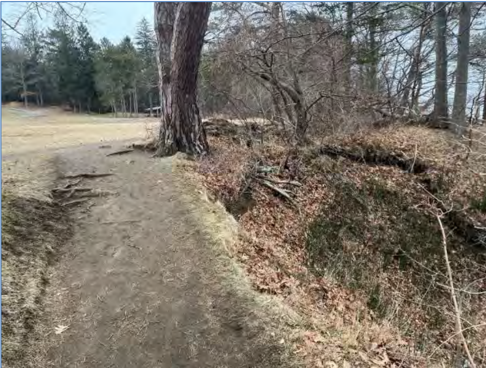
Fig. 14. Section of Trail Located at The Top of a Steep Coastal Slope
