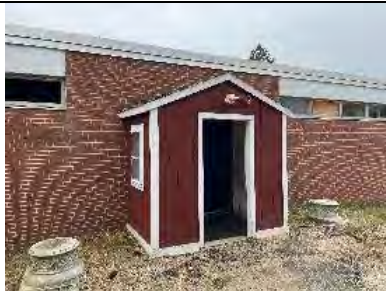
T-1-11 entry vestibule.
