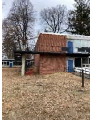
Canopy/overhang and exterior stair east side
