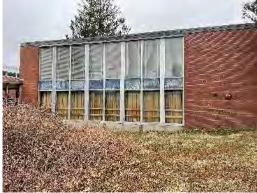
Aluminum curtainwall.
