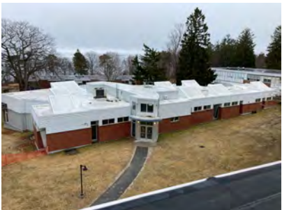
BREWSTER HALL: BUILDING H
