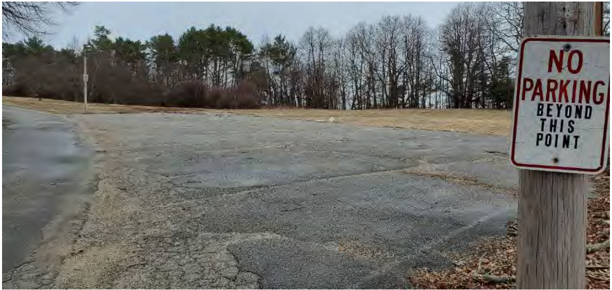
Photo 7: Athletic Field area parking lot
