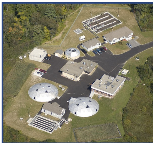
Falmouth's wastewater treatment facility on Clearwater Drive.
