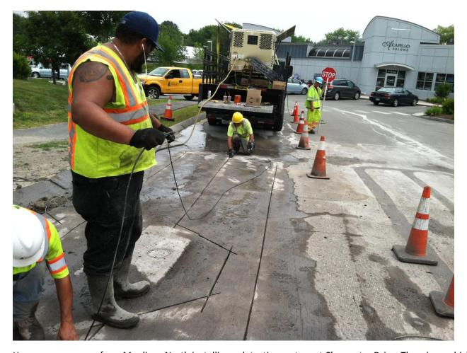
Here, we see a crew from Moulison North installing a detection system at Clearwater Drive. The wires, which are laid into a precisely-cut system of grooves in the asphalt, will use a magnetic field to sense waiting traffic.
