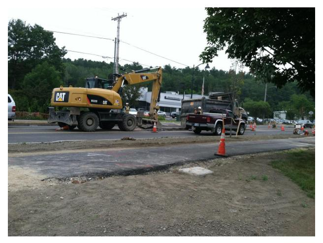
Pedestrian safety is a big consideration, and some crosswalks are being installed in areas between traffic signals. This is one such location, between the Morong dealership and the Morong service facility. We see a crew from Sargent Corporation removing pavement in the center of Route One. A curbing crew will install granite curbing this week; another crew will add cobbles inside the pavement, and the island will be deeply filled with loam. Attractive perennial plants will then be planted.
