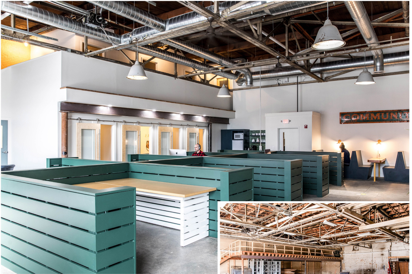
ABOVE | COWORKING STUDIO SPACE WITH CONSTRUCTION PROGRESS IMAGE OF SPACE PREVIOUSLY USED FOR CITY OF PORTLAND VEHICLE MAINTENANCE SHOP
