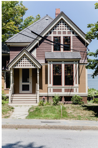
ABOVE | RESTORED EAST ELEVATION OF HOUSE, EL AND BARN
