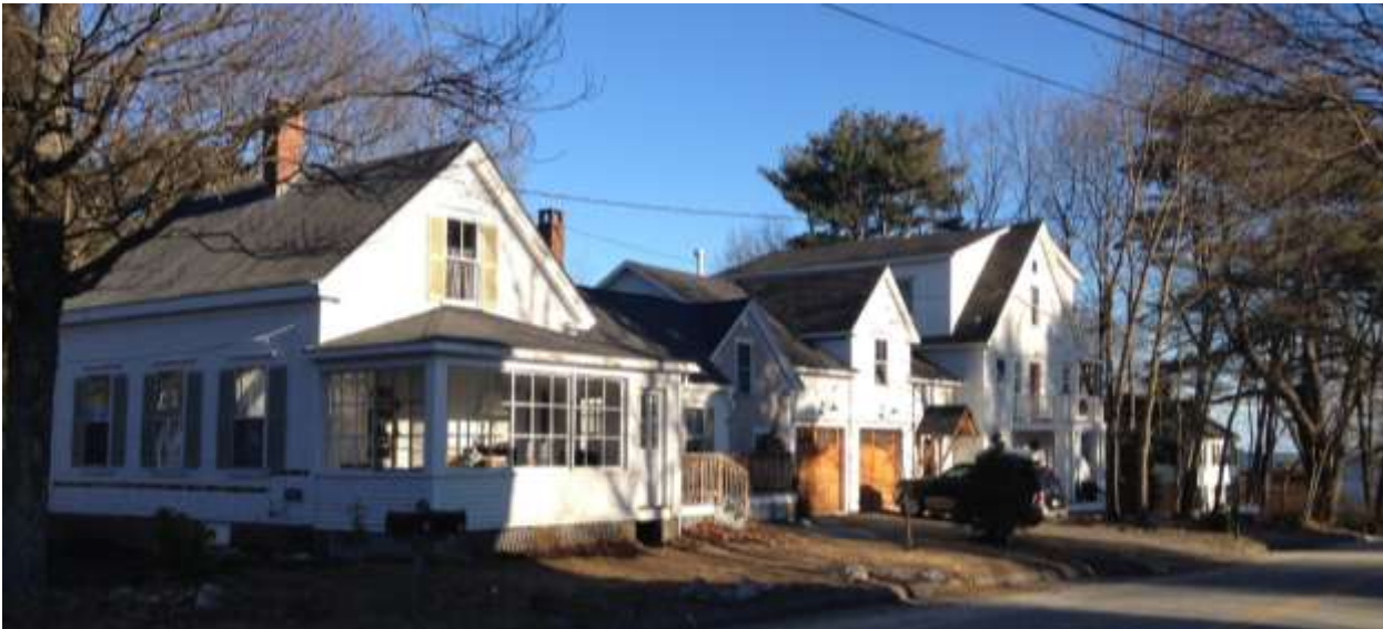
Figure 8: Town Landing Road
