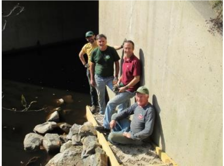
Photo 10 Volunteers work on a canoe launch to improve access to the East Branch Conservation Area.
