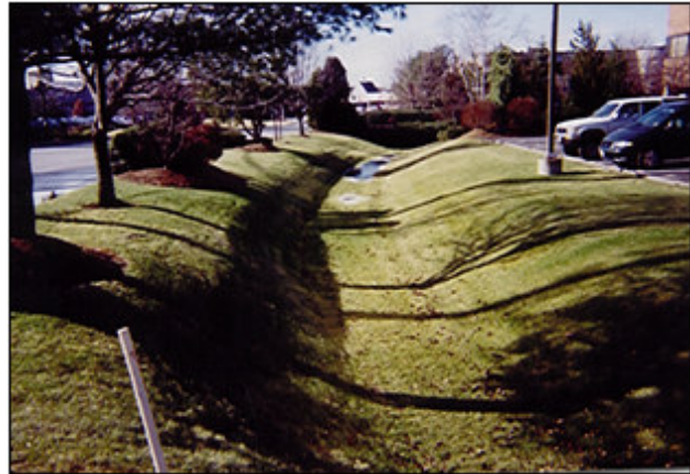
This dry swale is located in New Hampshire. It blends well with the landscaping and is low maintenance yet effective. It does have an overflow to the storm drain system that can be accessed once the water reaches more than halfway up the side slopes.
