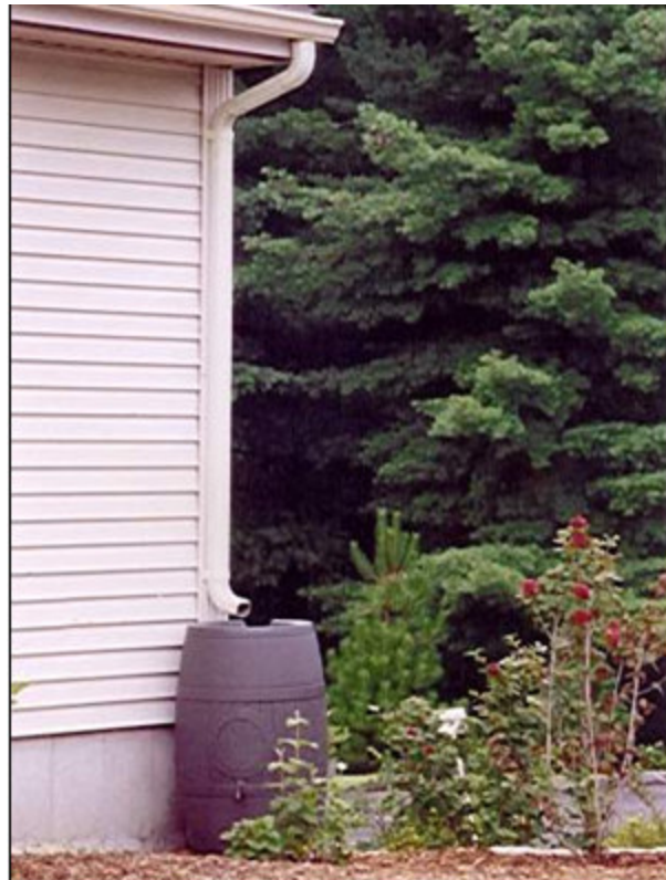
The above photo shows a rain barrel used to collect and store roof runoff for later use.
