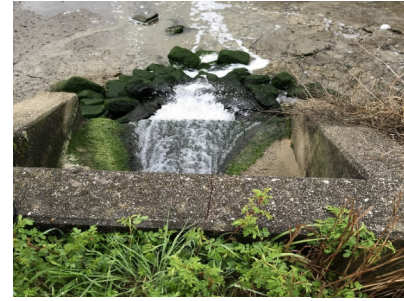
Outfall Pipe Headwall
