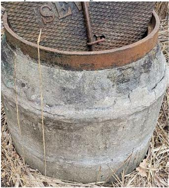
Manhole 67 Frame - Fracture
