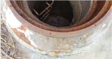
Manhole 63 Chimney Interior - Infiltration Dripper
