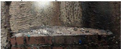
Manhole 39 Channel - Deposits Attached Grease
