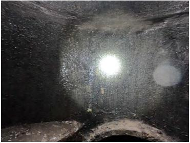
Chimney Interior - Infiltration Dripper
