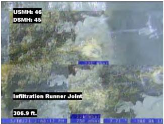
**46 - 45 Infiltration Dripper Joint**
