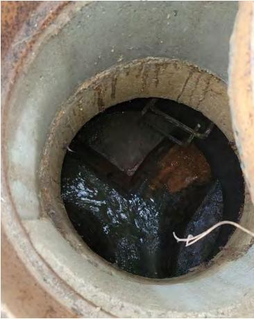
Stub Connection - Infiltration Dripper
